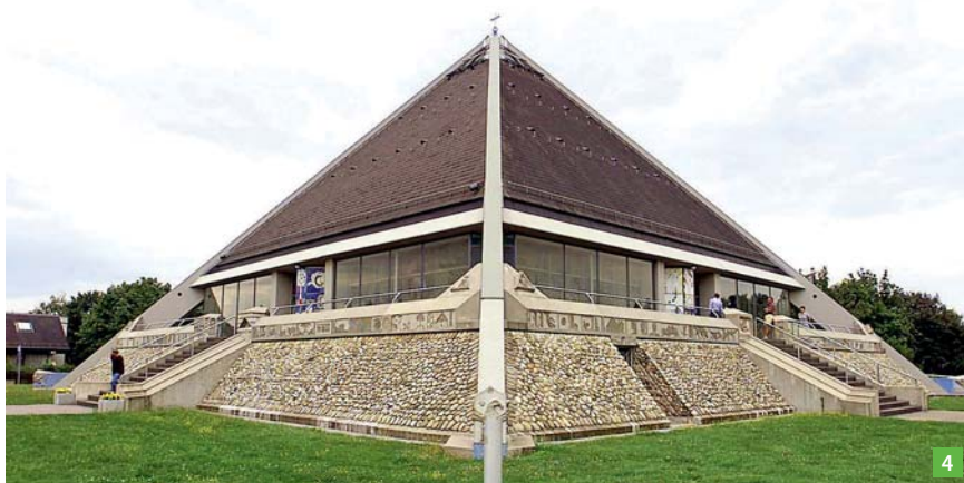
Foto: Ulli Deck/Picture Alliance
